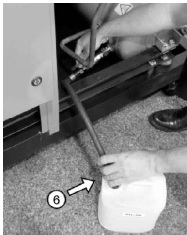
Fig. 6.11: Drain off old oil from oil/compressed air receiver
